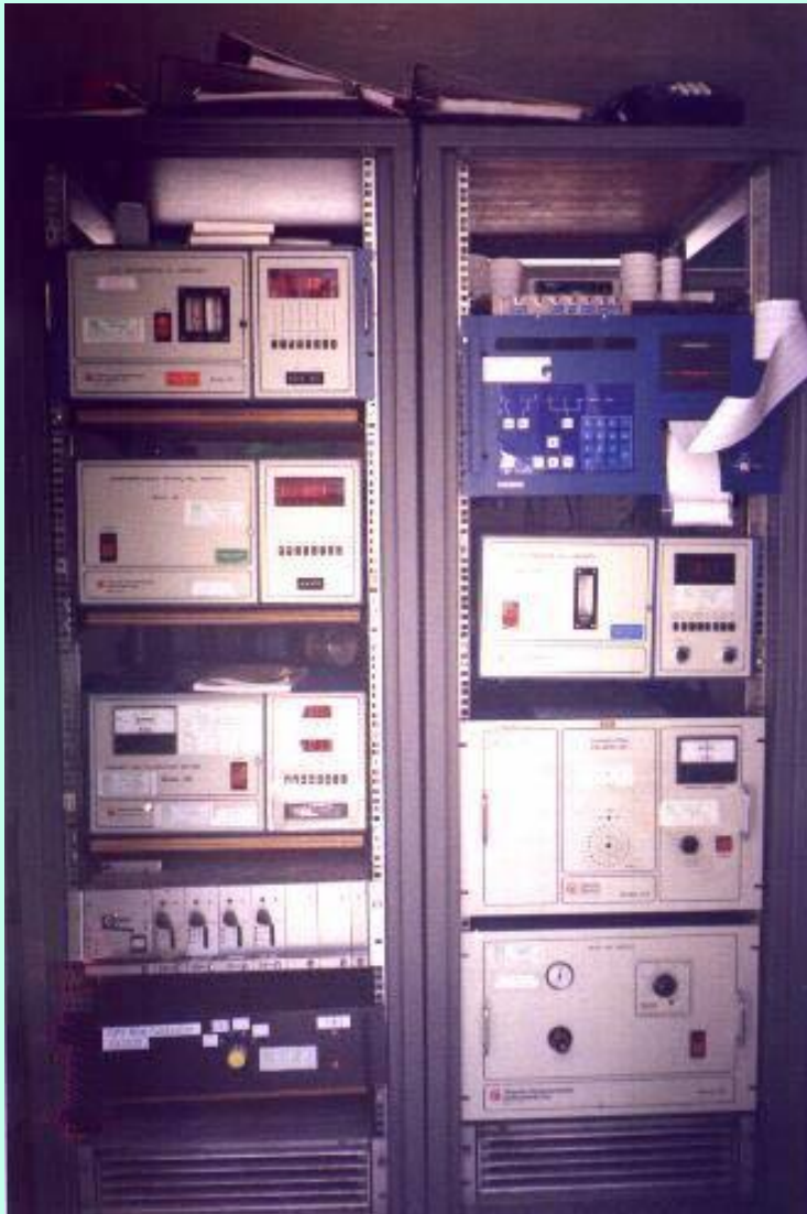
Gaseous pollutants analyzer
